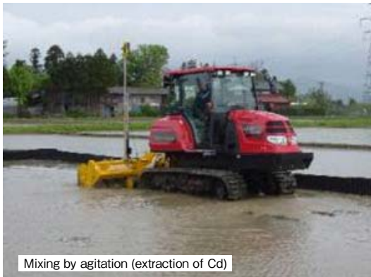
Fig. 3a Flow of the processes of chemical cleaning of paddy soil
